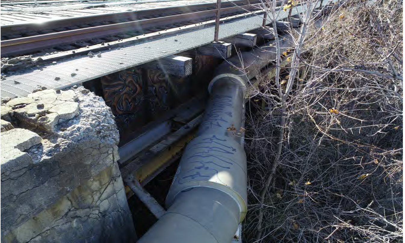
Jacketing along eastern bridge abutment, looking west
