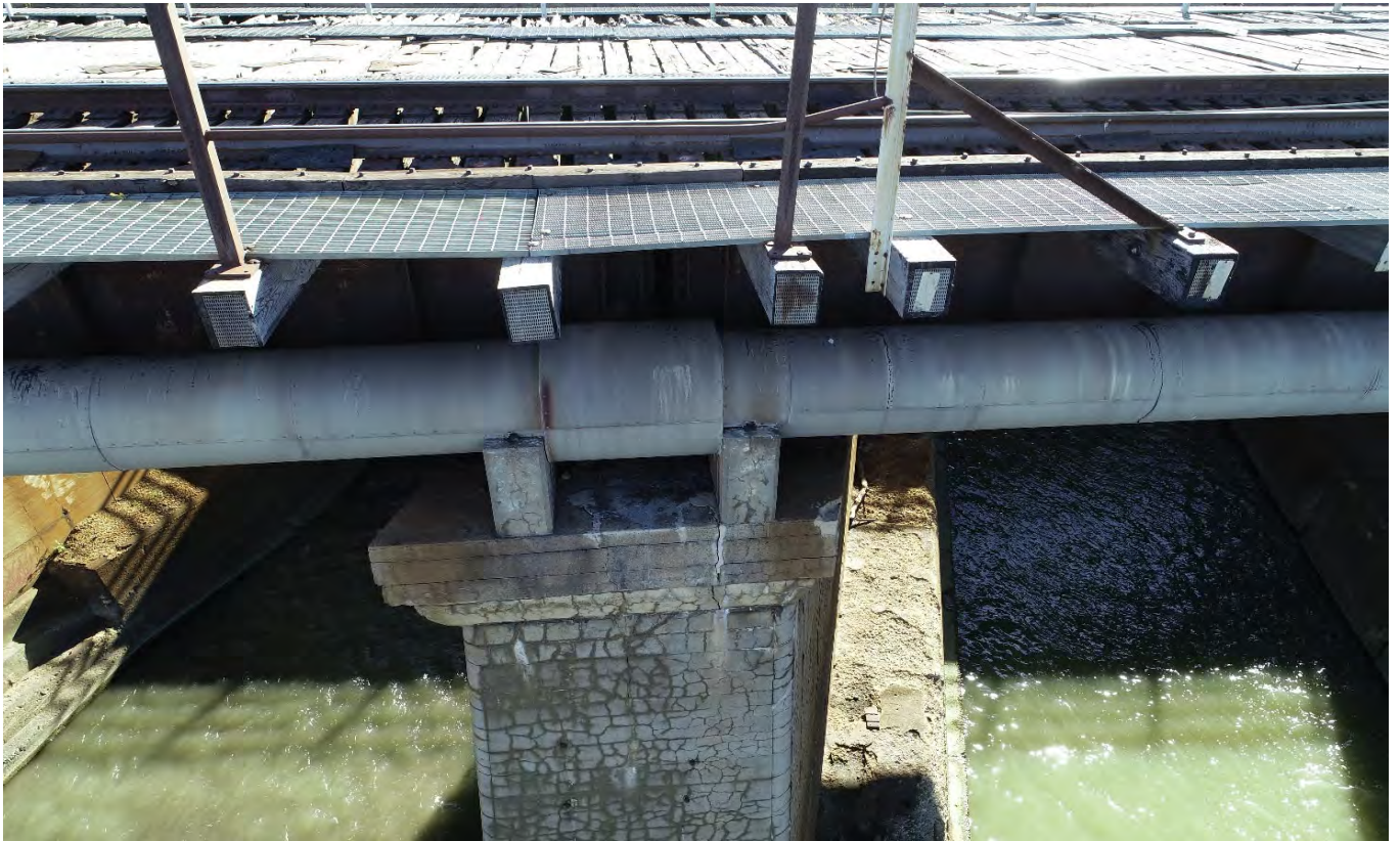
Pipe support at bridge pier and walkway looking south
