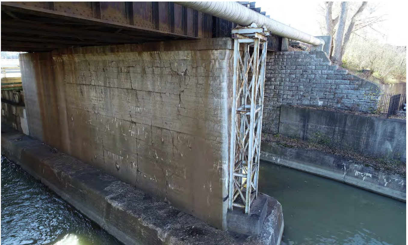
Steel support at east end of structure
