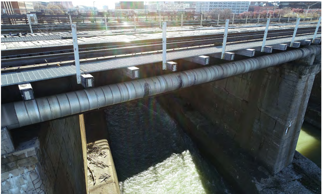
Pipe supported on bridge piers, looking south
