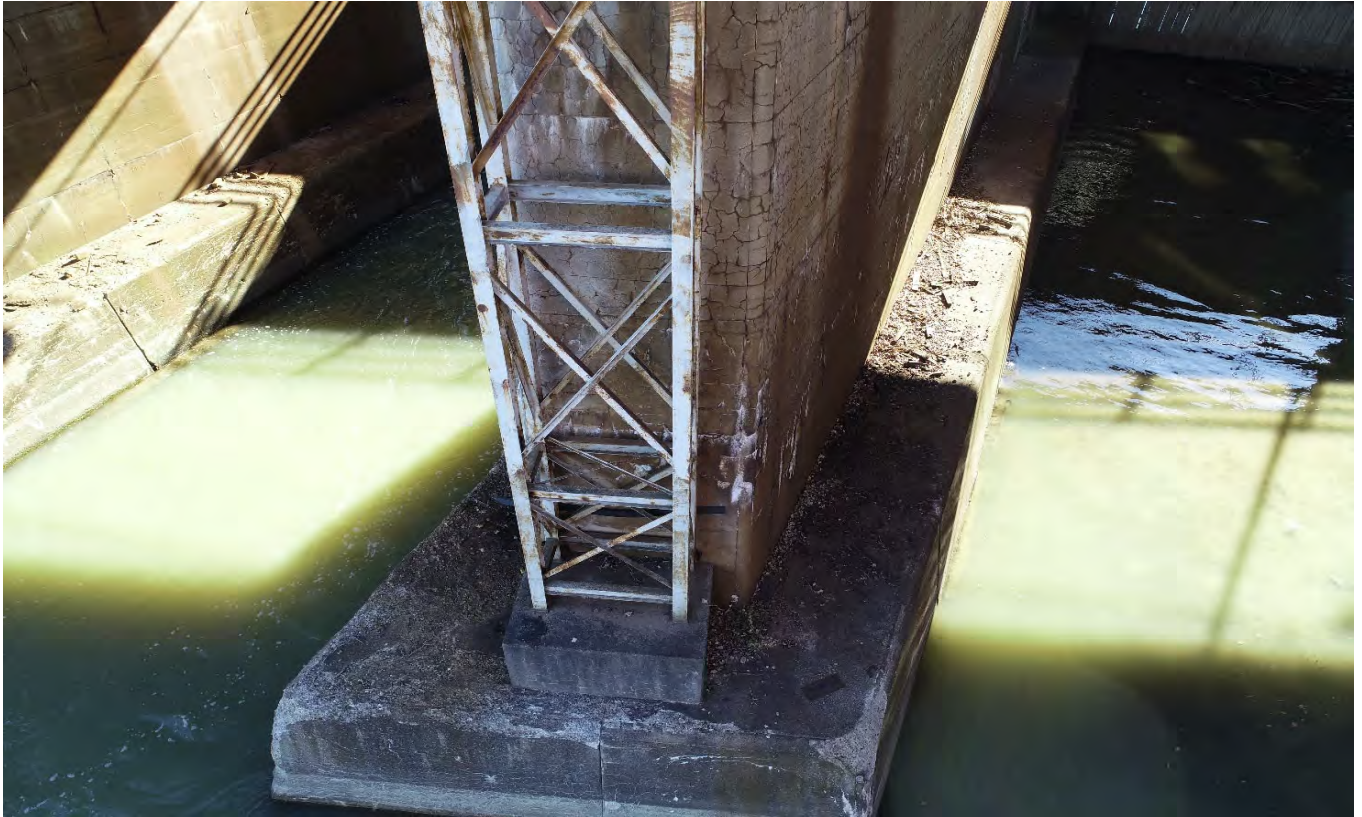
Bottom half of steel bridge support, east end
