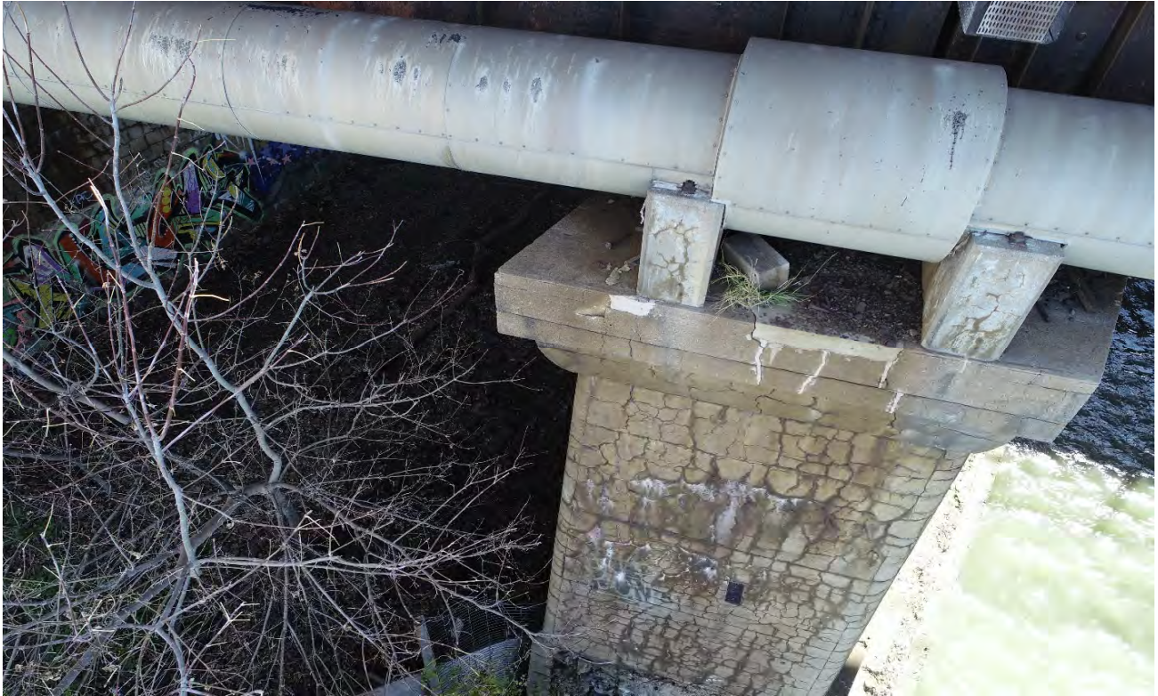
Pipe jacketing at bridge pier looking south
