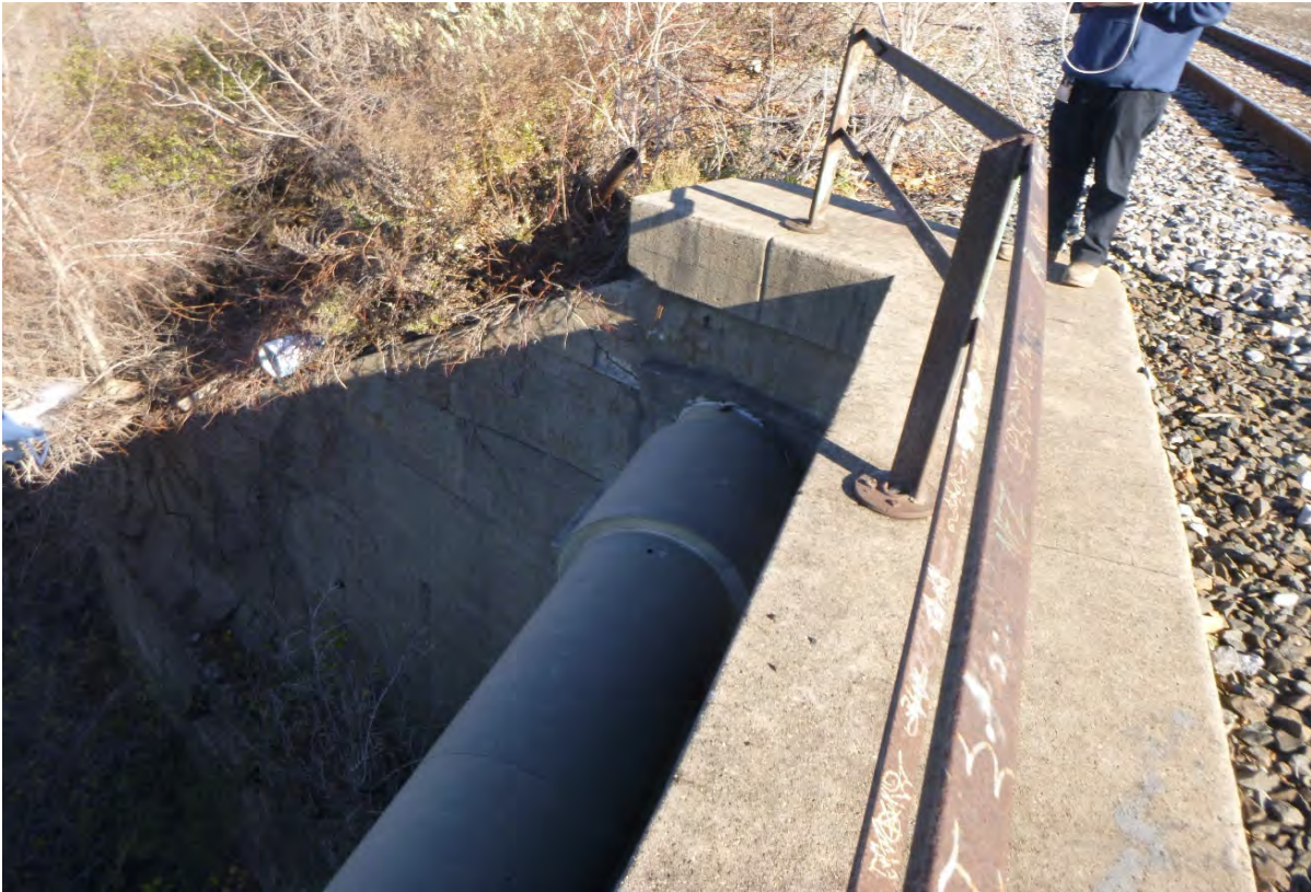
Pipe penetration at east abutment
