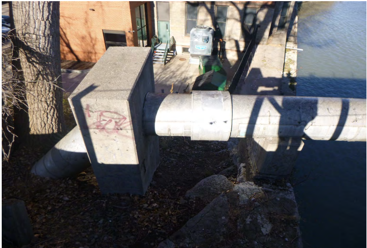
Pipe penetration at west abutment
