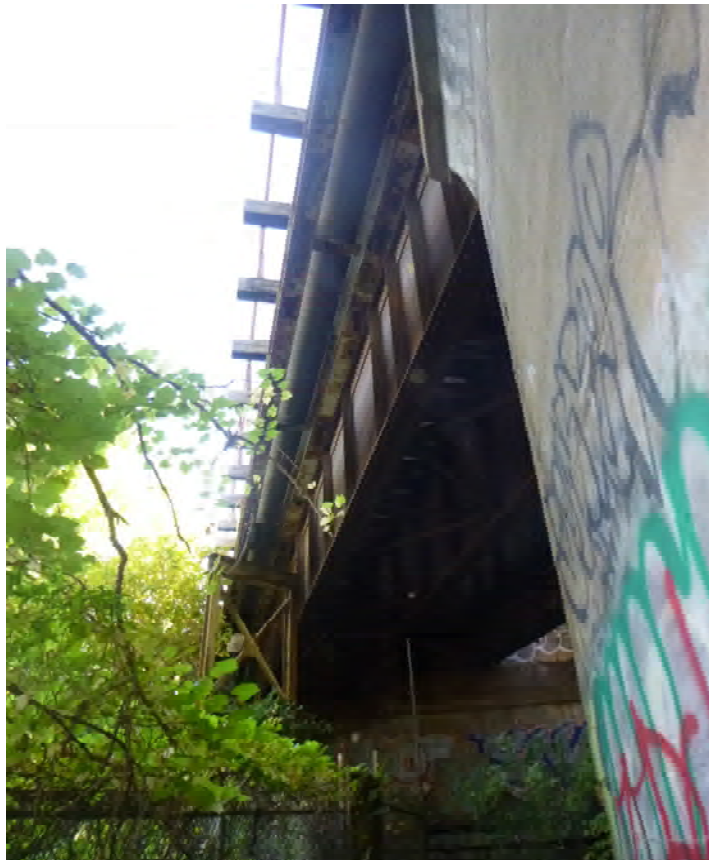
Underside of water main looking east between steel support and bridge pier (accessed from underside of CSX bridge)
