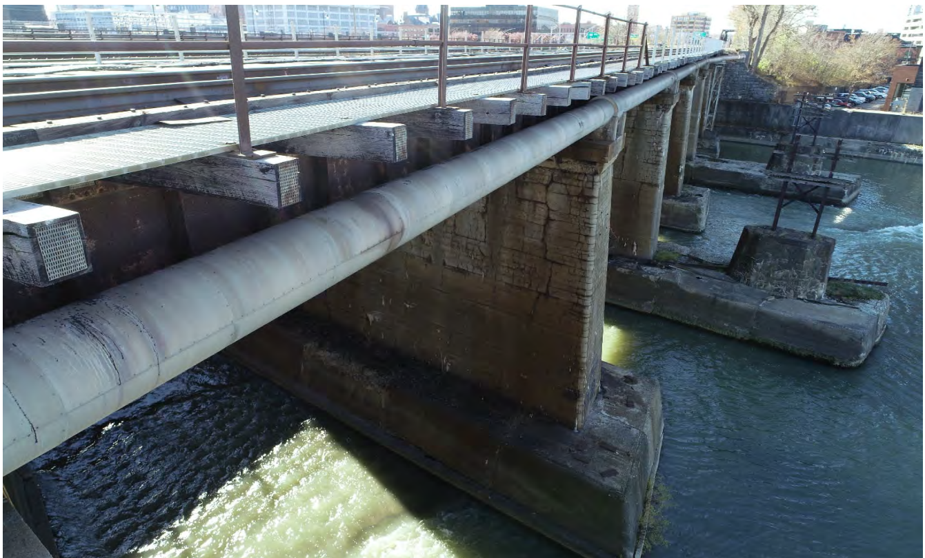
Pipe jacketing and supports looking south west
