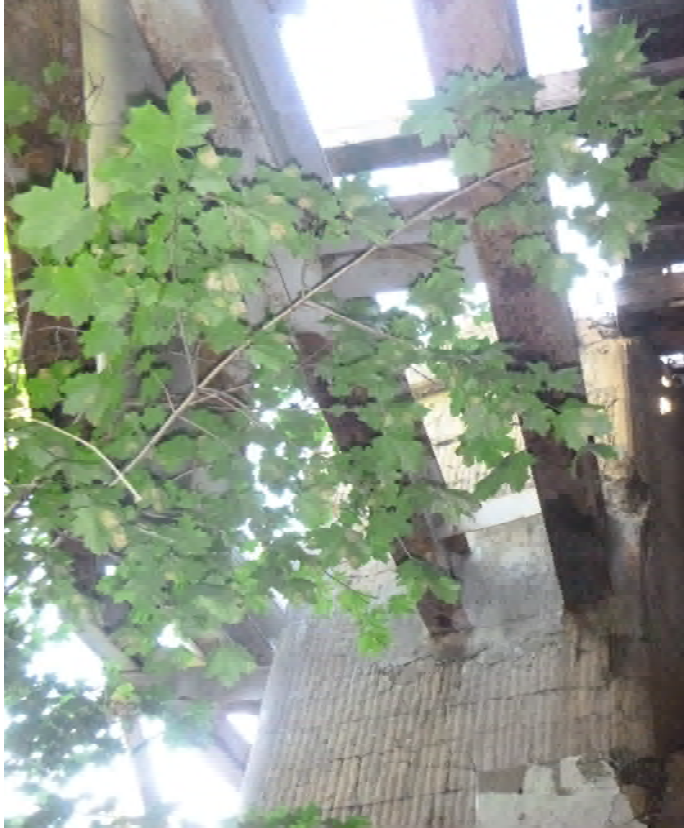
Steel supports attached to eastern bridge abutment (accessed from underside of CSX bridge)
