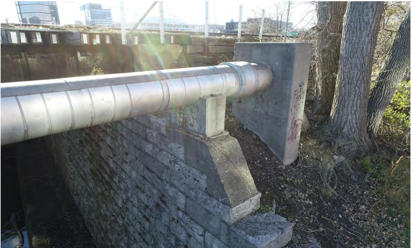
Western abutment - at CSX bridge abutment wall
