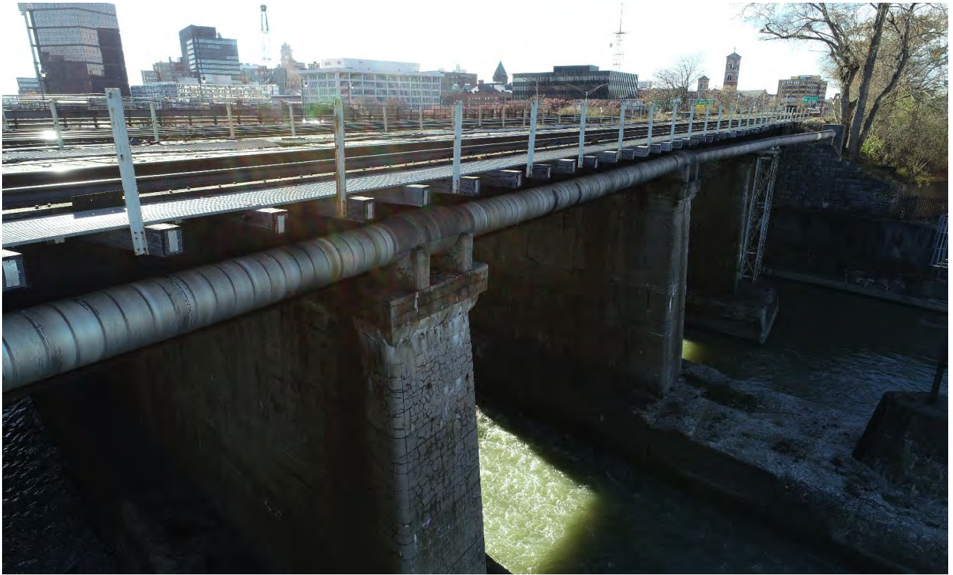
Pipe support on northern side of bridge, looking south west
