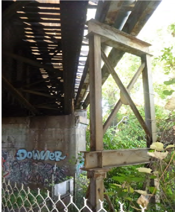
Steel support at eastern end of bridge abutment (accessed from underside of CSX bridge)
