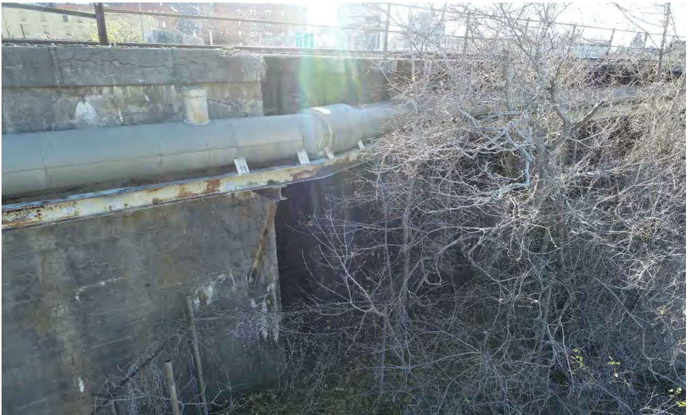
Pipe jacketing and air release on eastern end of bridge
