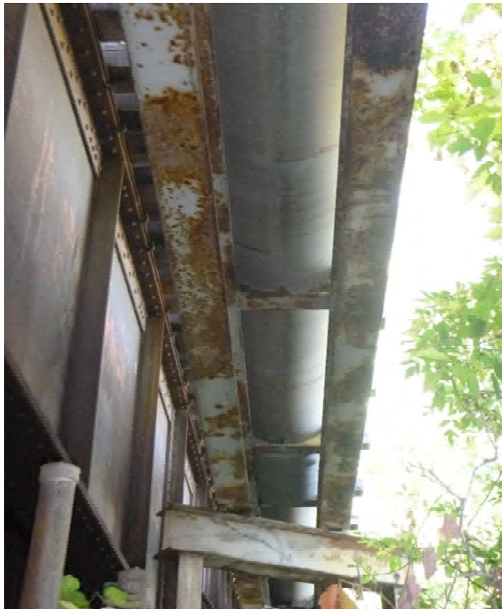
Underside of watermain supported on steel I-beams looking west (accessed from underside of CSX bridge)
