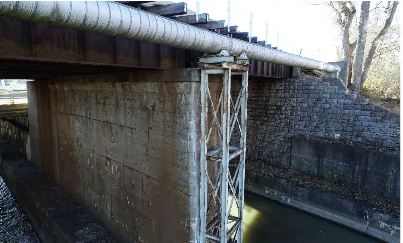
Steel support at east end of structure
