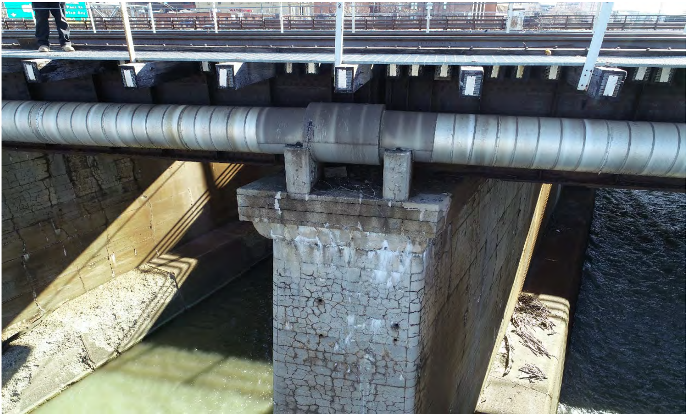
Jacketing on bridge pier looking south
