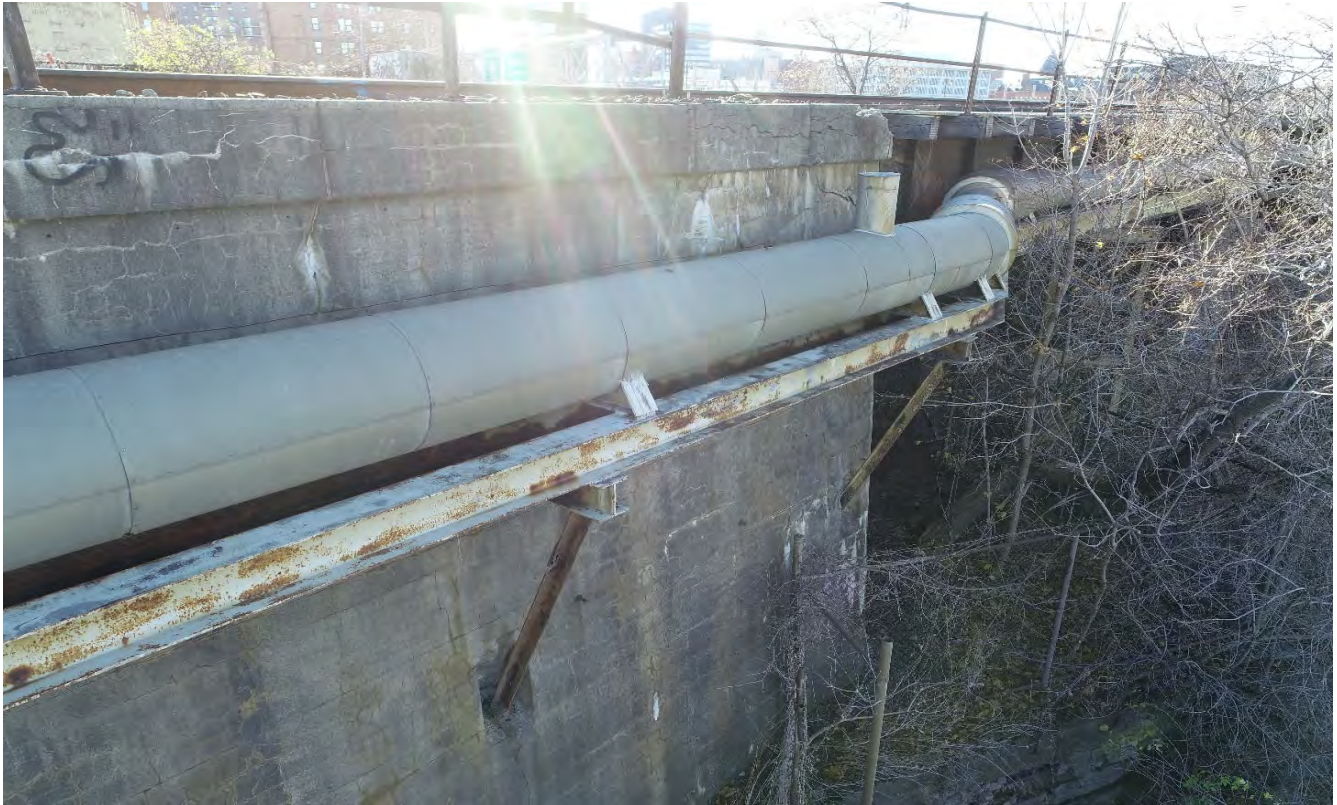
Pipe jacketing on steel supports affixed to east abutment wall, looking south west
