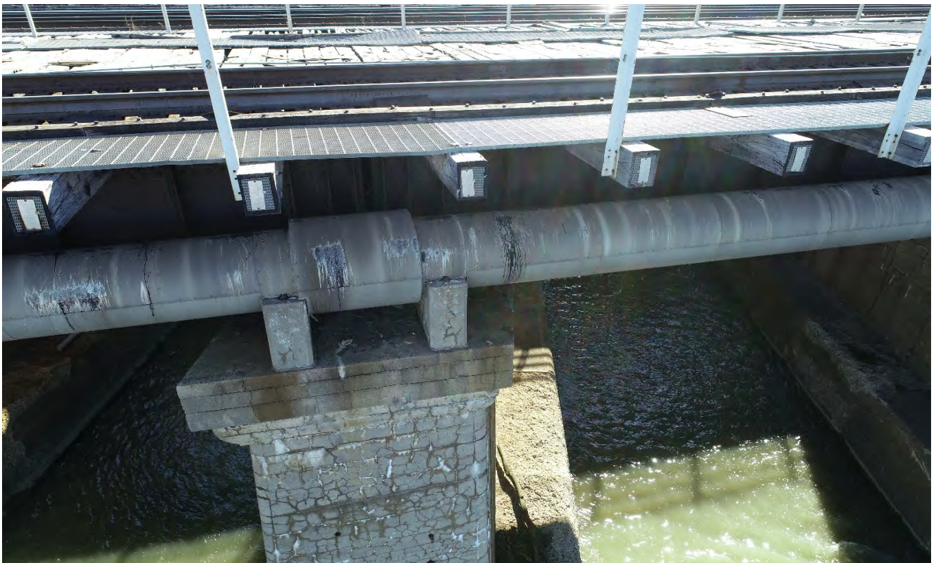
Pipe jacking and support at pier looking south
