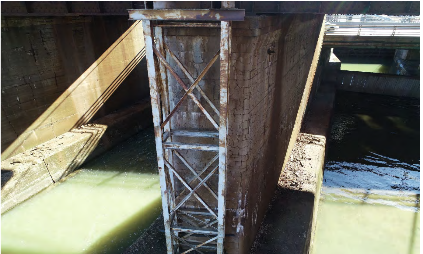
Top half of steel bridge support, east end
