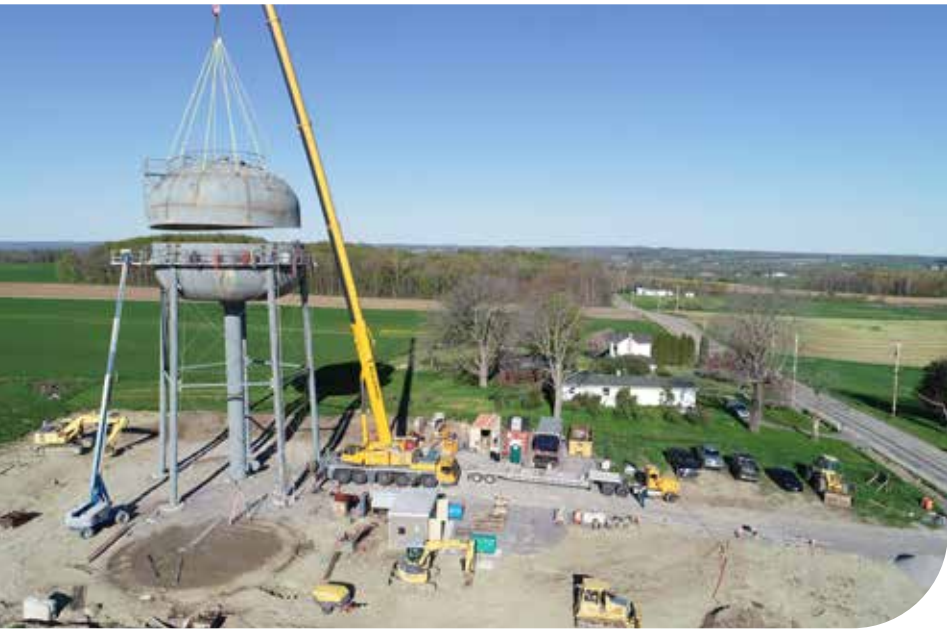
The Better Half A crane slowly lowers the top half of a new water tower tank into place in the Genesee County town of Pavilion, part of MCWA’s commitment to invest in water infrastructure improvements.
